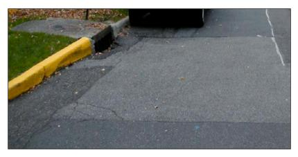
these conditions are caused by age and harsh winter conditions, and are in immediate need of repair. Work would include concrete curbing, and repair/replacement of concrete sidewalk and asphalt road.
