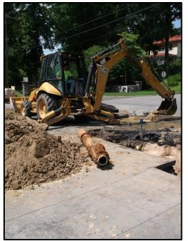
includes the upgrade of the existing water vault. Previously, the water main entering the vault was restricted before it continued onto the distribution system. This severely limited the flow and pressure of the water main and prevented adequate water distribution for the entire campus. This phase was completed in January 2013.
